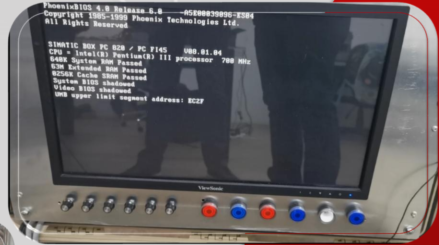
Upgrade de sistema PLC
